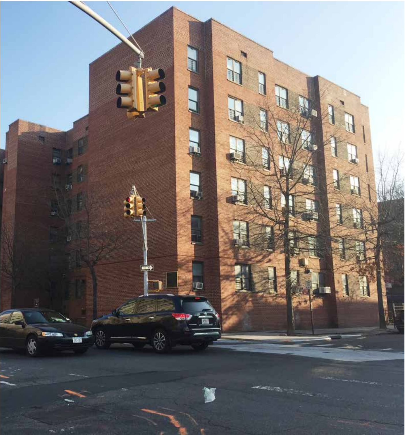
NYCHA Warren Street Houses
