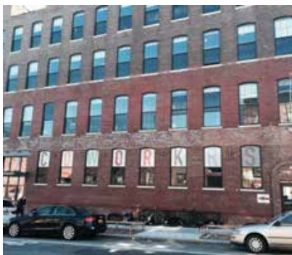
68 3rd Street, recently renovated for offices
