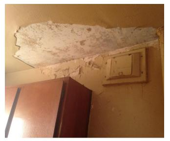
As seen from the photos above the problem of chipped paint is a serious issue. This degree of deterioration is a valid reason for maintenance to address a resident's problems, particularly in light of NYCHA's lead-paint neglect.
