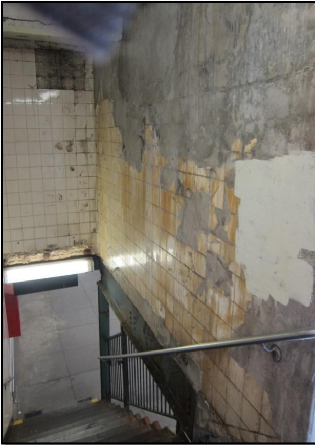
Figure 3: Example of Deteriorating Walls at Rector Street (R)
