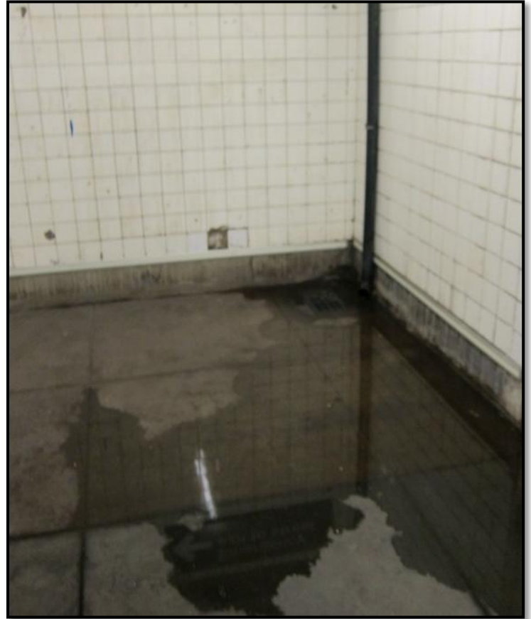
Figure 4: Example of Ponding in Borough Hall (2/3)
