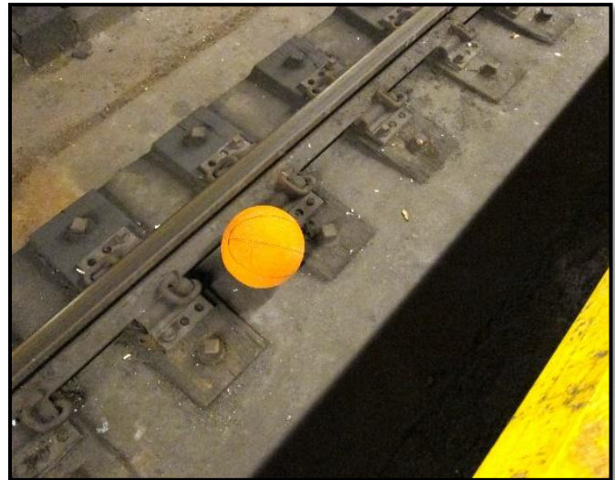
Figure 1: Basketball on the tracks at Chambers Street (J/Z)
