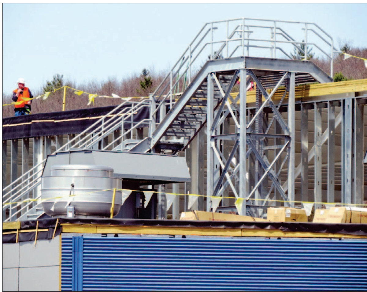
Construction is underway on a 94,000-square-foot expansion of Corning Inc.'s heavy duty diesel plant in Erwin. Company officials credited strong manufacturing performance at the plant with helping to drive a sharp increase in profitability in the Environmental Technologies business. DERRICK EK/THE LEADER
