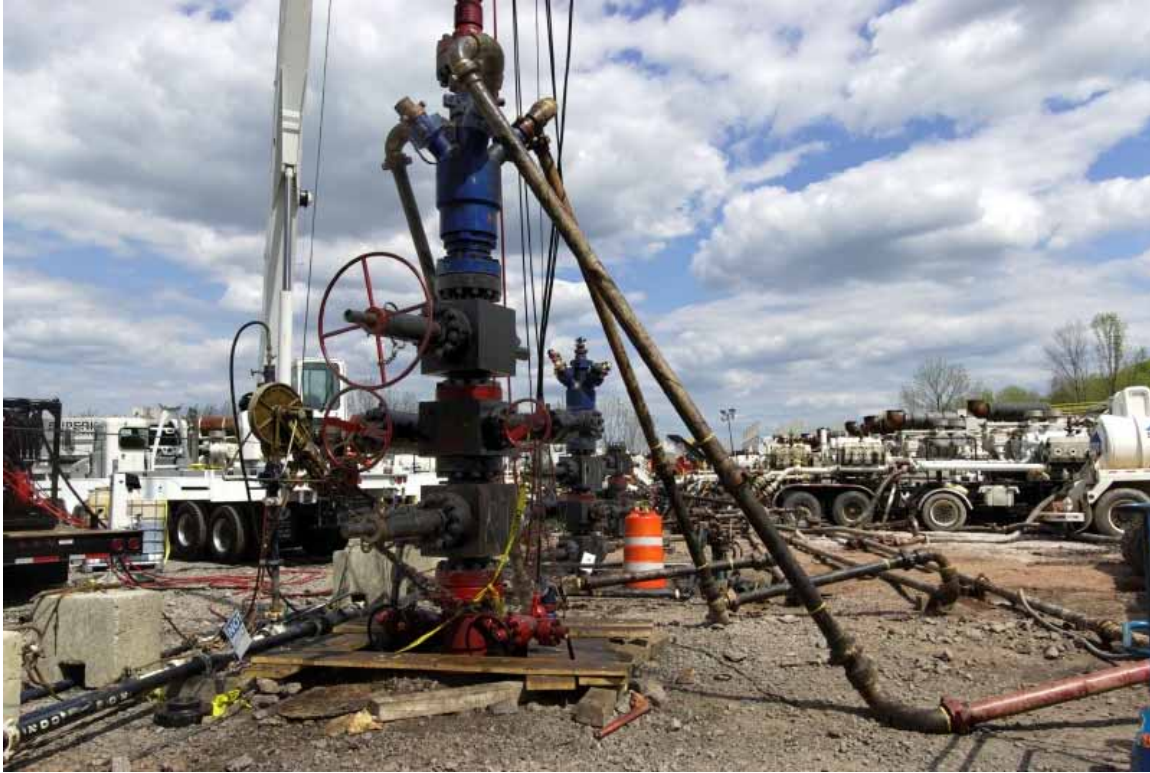
Photo 5.24 - Three Fortuna Energy wells being prepared for hydraulic fracturing, with 10,000 psi well head and goat head attached to lines. Troy PA. Source: NYS DEC 2009
