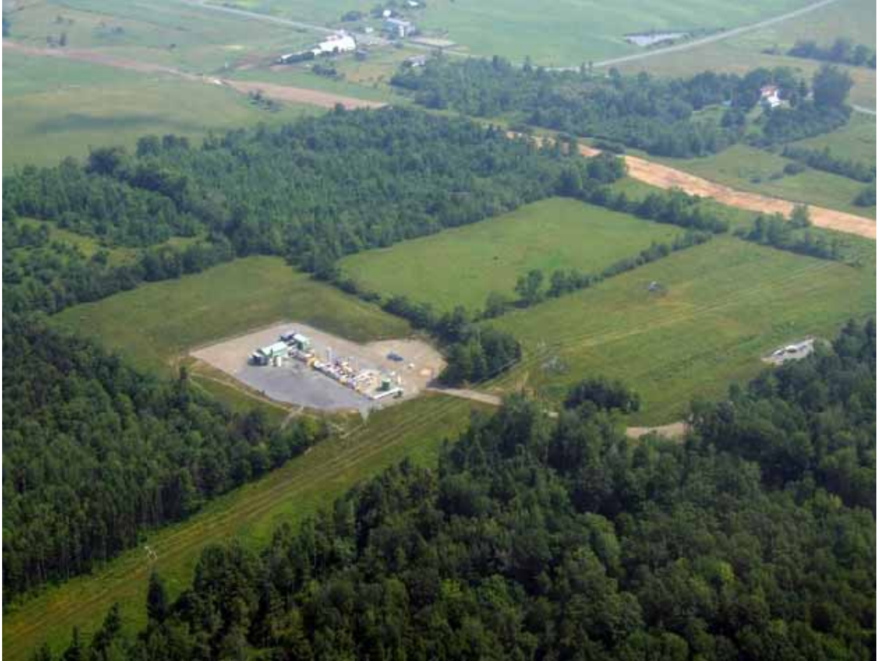
Photo 5.27 - Pipeline Compressor in New York. Source: Fortuna Energy
