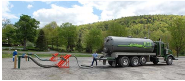
Photos 5.20 a & b Fortuna SRBC-approved Chemung River water withdrawal facility, Towanda PA. Source:
