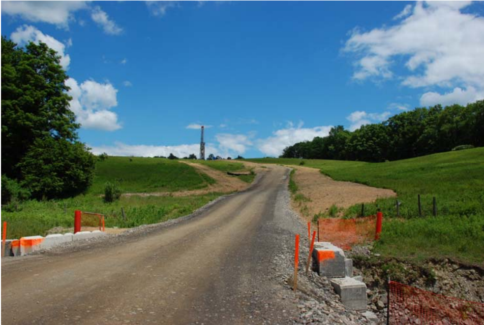
Photo 5.1 Access road and erosion/sedimentation controls, Salo 1, Barton, Tioga County NY. Photo taken during drilling phase. This access road is approximately 1,4000 feet long. Road width averages 22 feet wide, 28 feet wide at creek crossing (foreground). Width including drainage ditches is approximately 27 feet. Source: NYS DEC 2007.
