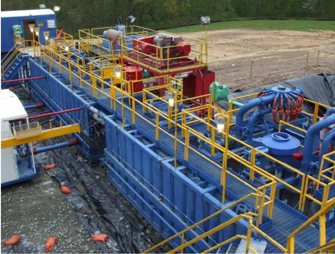
Photo 5.16 - Drilling rig mud system (blue tanks)
