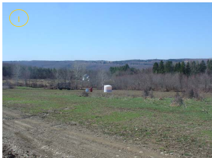
Photo 5.9 The above map shows a portion of the Chautauqua County map, near Gerry. Well #1 (API Hole number 25468) shown in the photo to the right was drilled and completed for production in 2008 to a total depth of 4,095 feet. Of the other 47 Medina gas wells shown above, the nearest is approximately 1,600 feet to the north.
