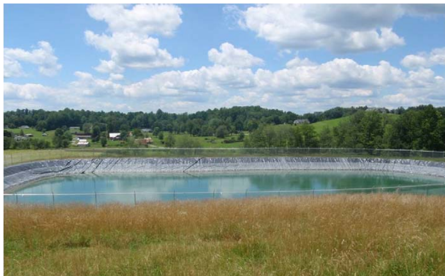
Photo 5.23 Construction of freshwater impoundment in Upshur Co. WV. Source: Chesapeake Energy
