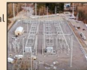
115 kV Substation Rebuild (Big Tree)
