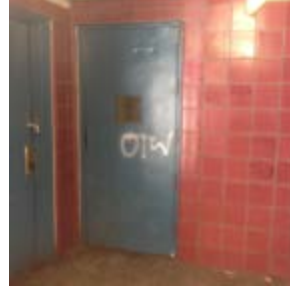
A gang tag on an exterior door in Wagner Houses.
