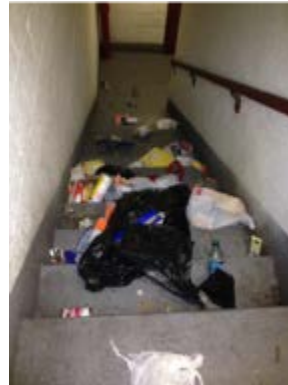
Debris clogs this stairwell in Wagner Houses, rendering an escape difficult at least.
