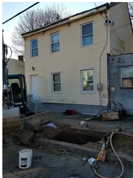
Figure 6 – An LSL replacement in Newburgh funded by DOH’s LSLRP
