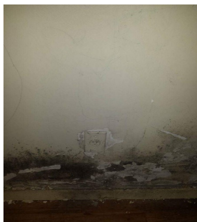
Mold covers the wall of a Bronx NYCHA apartment (2017).
