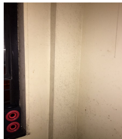
Black mold creeps up the wall of a Bronx NYCHA Apartment (2017).
