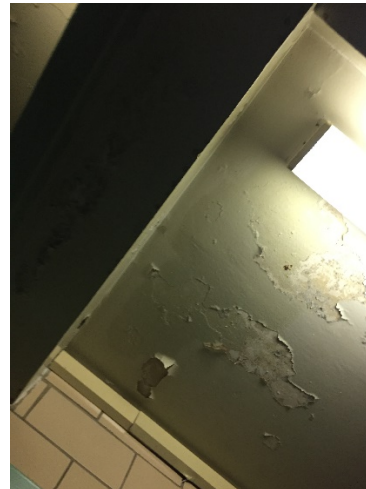
Paint is crumbling off of a hallway ceiling from what looks to be a leak. Mold is also evident (2017).
