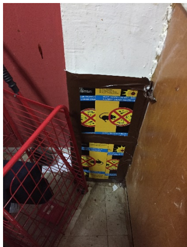
Cardboard and tape is used to cover exposed wall (2017).
