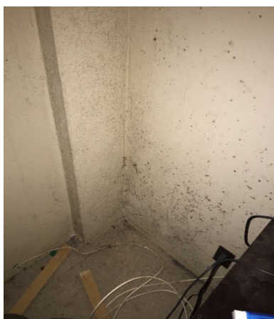
A severe case of black mold in a NYCHA apartment (2017).
